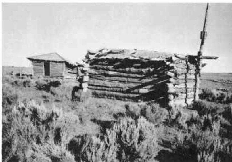
Fig. 13. Homestead of Vern McDonald on West Boulder five miles southeast of Monticello in Section 34, Township 33 south Range 24 east. Patent was issued August 14, 1923. The first house is made from pinyon logs and the second is made from sawed timber.
