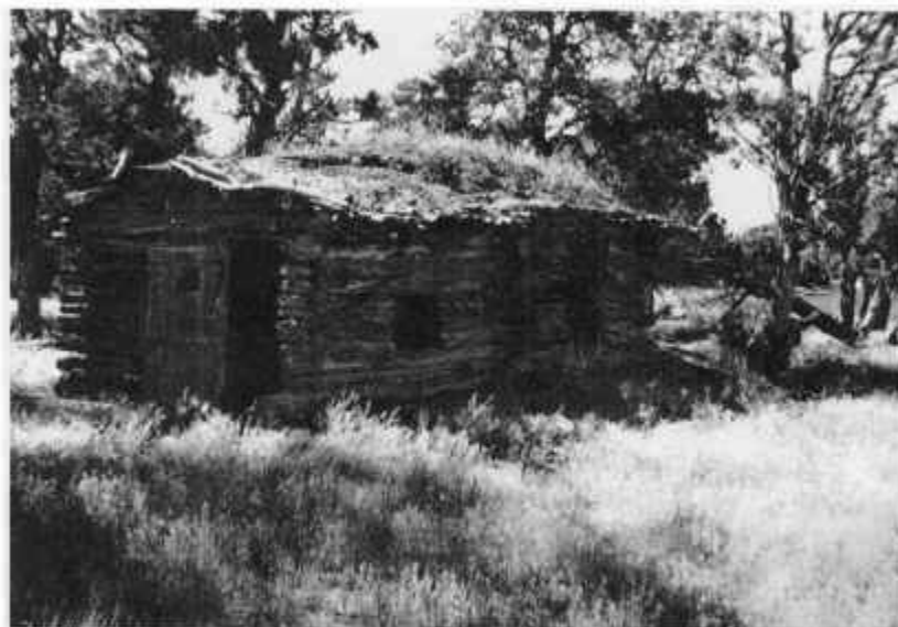
Fig. 14. Log house on Pearson Point made from juniper logs. Occupied by John P. Mansfield until the late 1930s.
